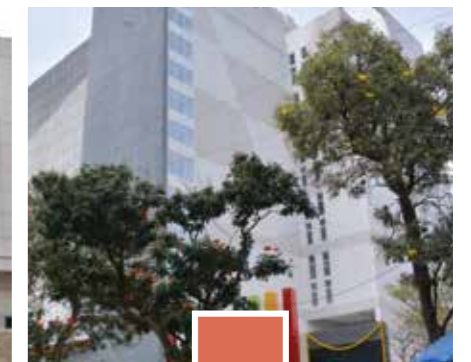
STT Data Center, Bengaluru
