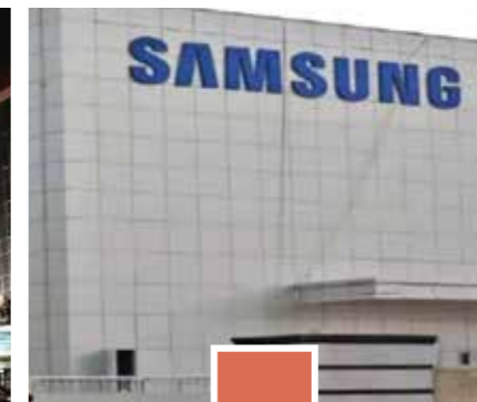
Samsung Manufacturing Facility, Delhi
